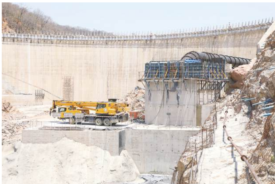
Lake Gwayi-Shangani requires US$48 million to complete the dam wall
